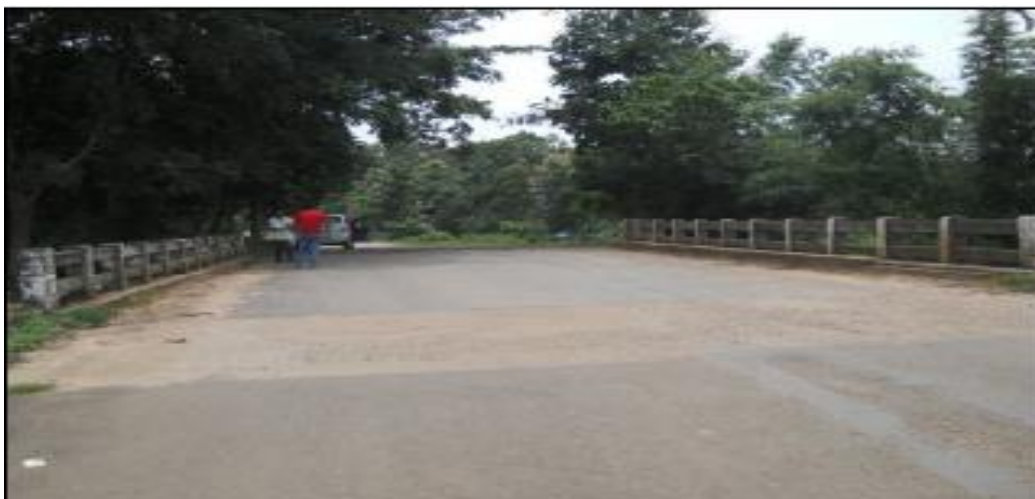
Figure 7: image of existing major bridge at chainage 12+400km
